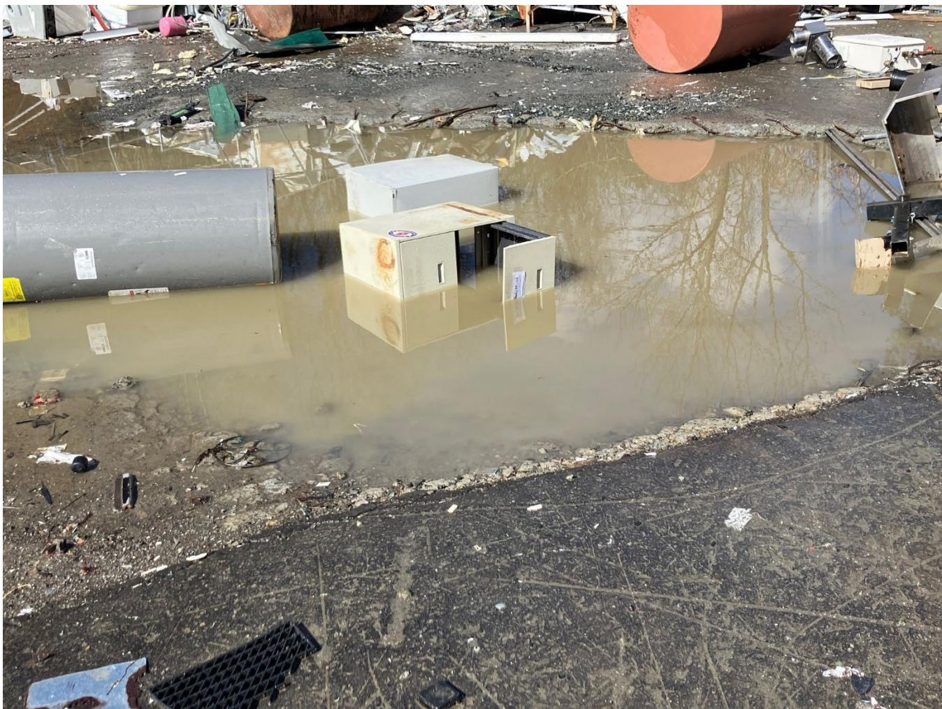
ABOVE: One of two areas in the current scrap metal pad that has degraded enough to hold water. Exposed rebar is also visible along the top of the 'lake'.
